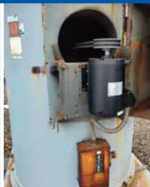
Replacement of welding exhaust fan
