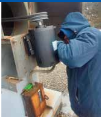
Replacement of welding exhaust fan
