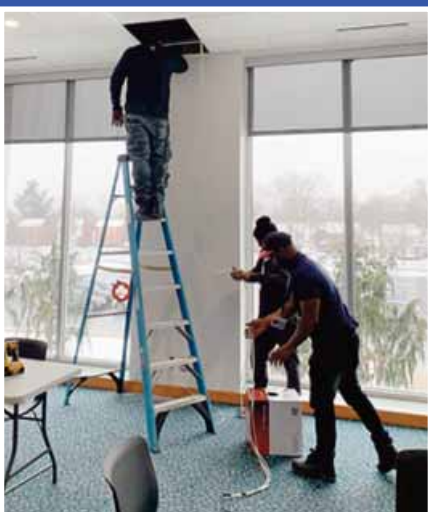
Installation of new data lines in the Culinary Arts and Hospitality Center at the Northwest Campus.
