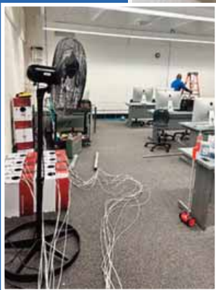
Wiring upgrades to MAC Lab
