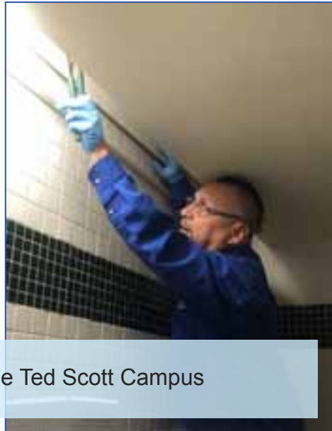
Replacing the light fixtures throughout the Ted Scott Campus
