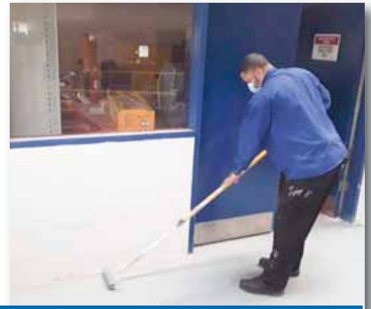
Painting HVAC Sheet Metal Lab
