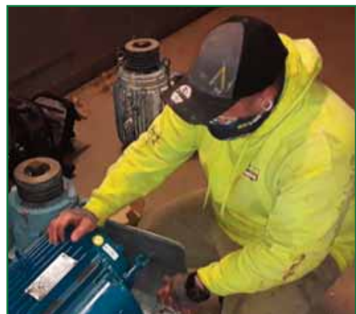
HVAC Cooling Tower Motor Repair
