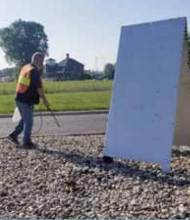
Install Hose Reel
