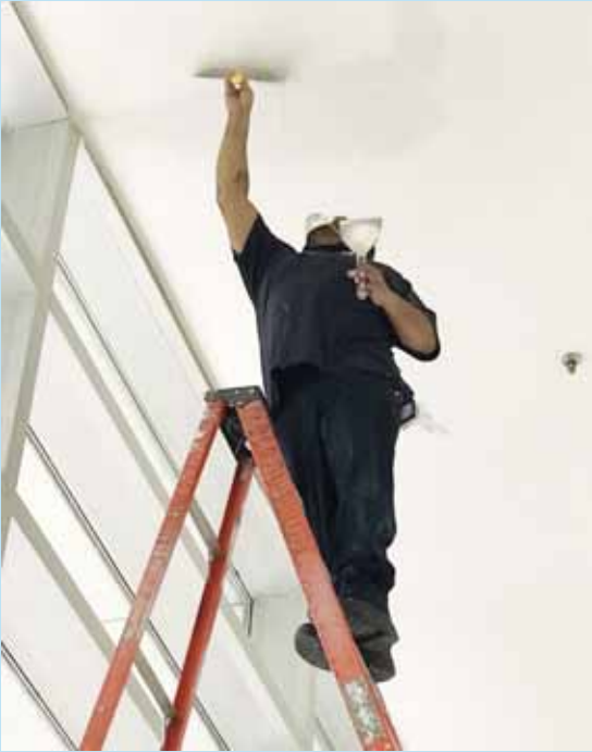
Wall Repair and Patch Work Project Eastern Campus
