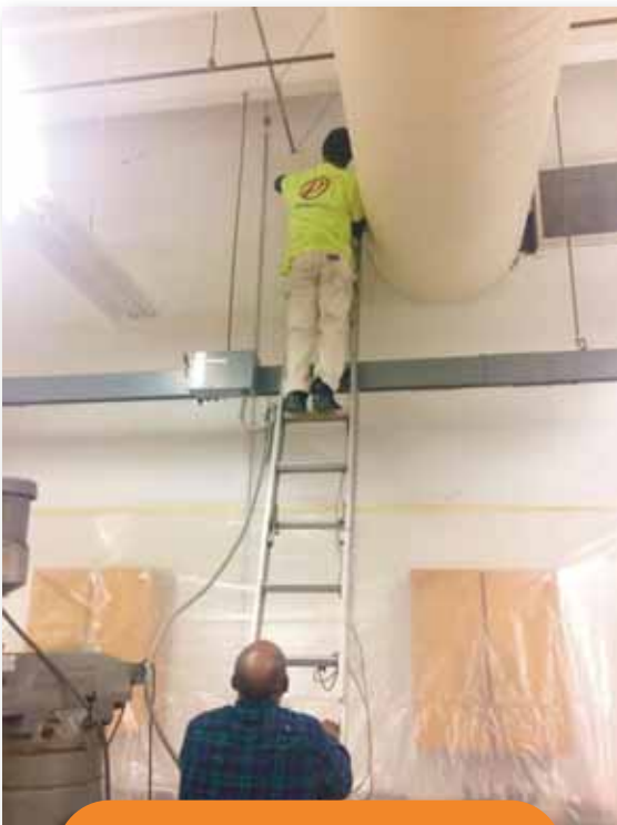
Eastern Campus Painting Project
