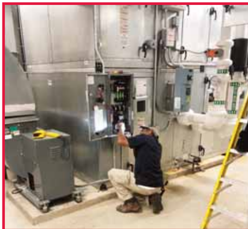
Northwest Campus Equipment Inspection and Repairs
