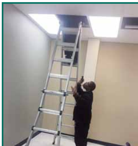
Northwest Campus Lighting Inspection and Repairs
