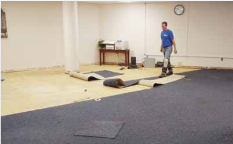
Downtown Campus Carpet Installation
