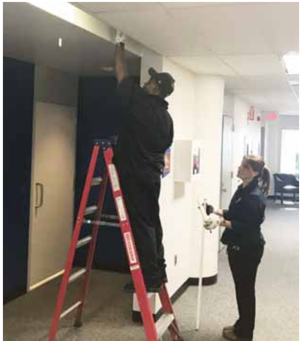
District Office General Repair
