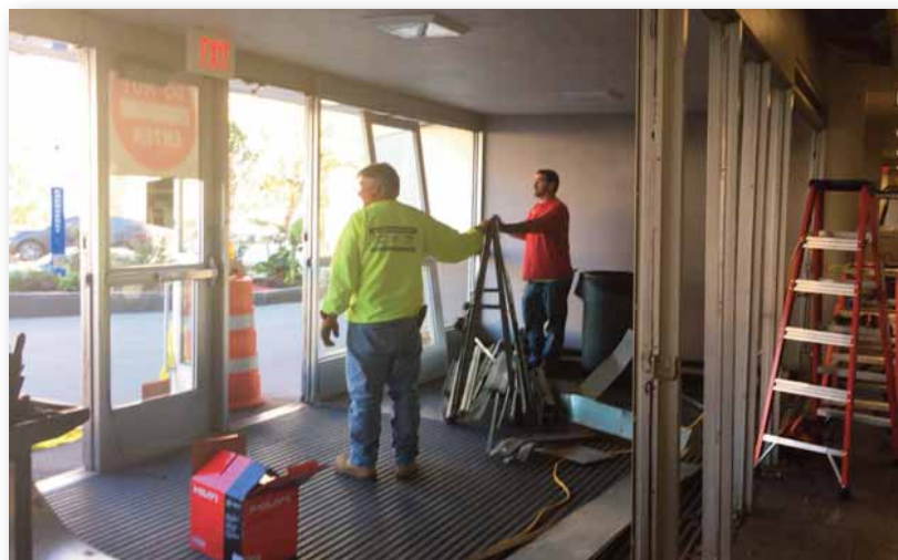
District Office Vestibule Renovation
