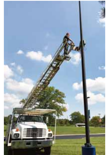
Eastern Campus Security Camera Repairs
