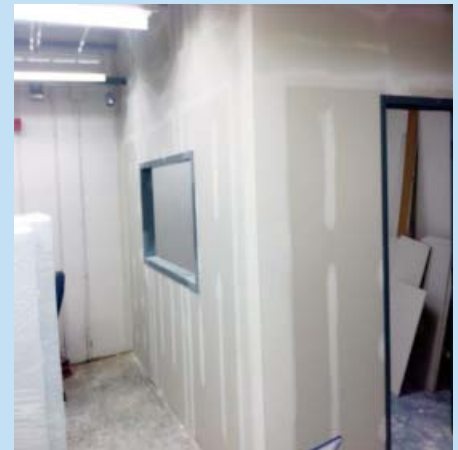
Police Authority Station
