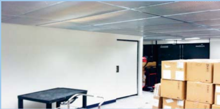
Installation of ceiling tiles
