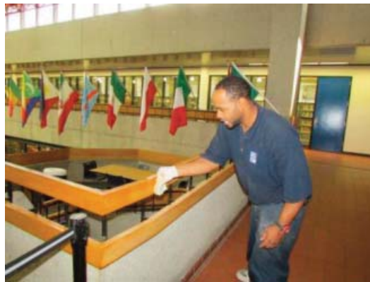
Downtown Campus Refinishing Oak Stair Rail
