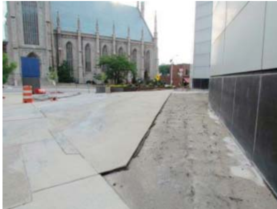
District Office Concrete Makeover
