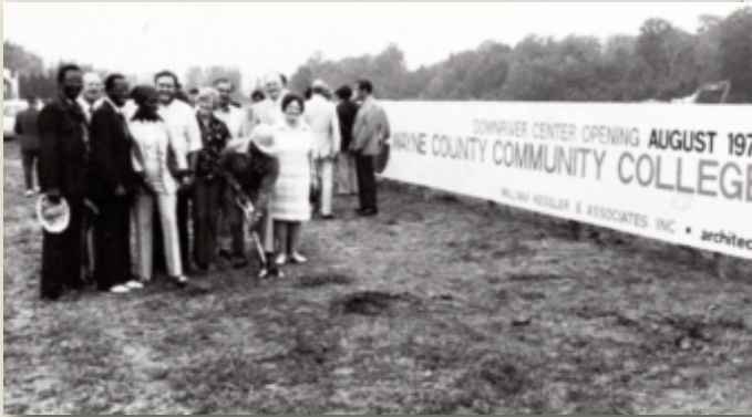
Groundbreaking for the Downriver Campus August 1978
