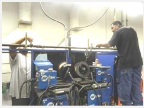
Replacement of compressor
