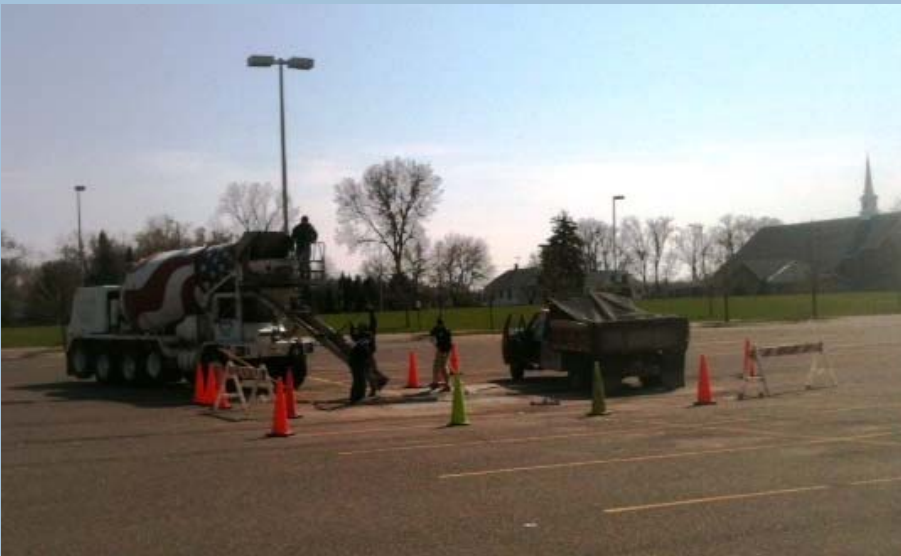
West Parking Lot Storm Sewer Repair at the Downriver Campus
