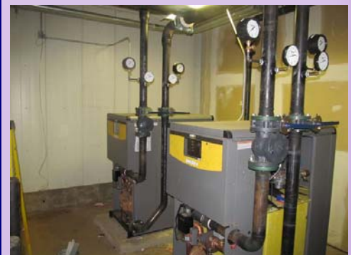
Mechanical renovation Continues at the District Office
