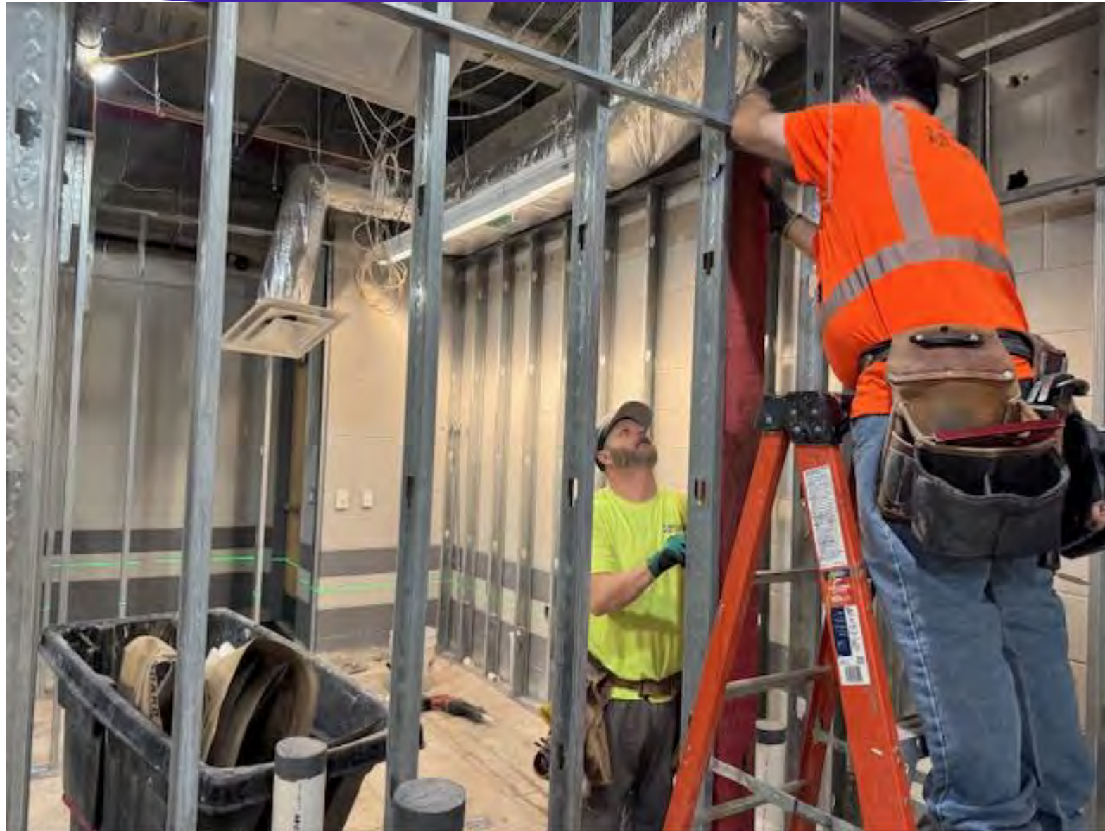
► Locker Room Renovation Project
