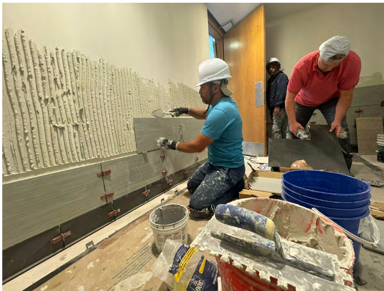
► Restrooms Renovation Project
