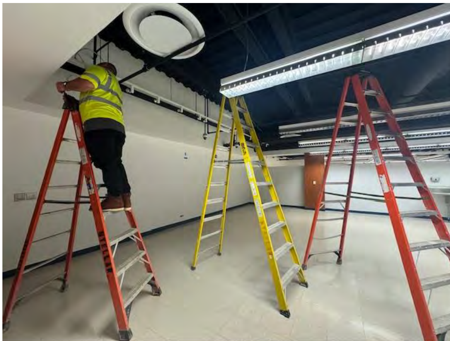
► Nursing Lab Renovation Project
