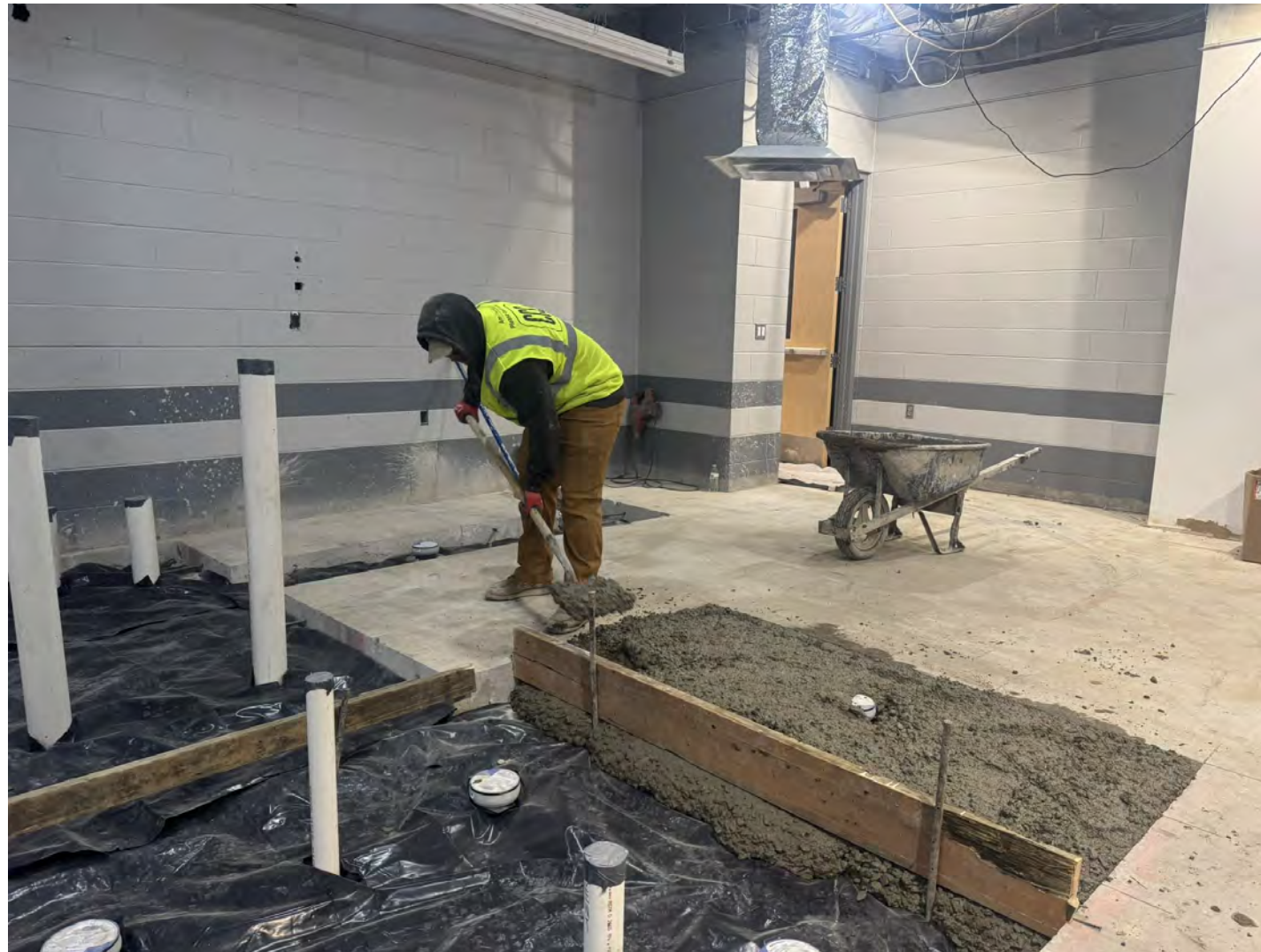
► Locker Room Renovation Project
