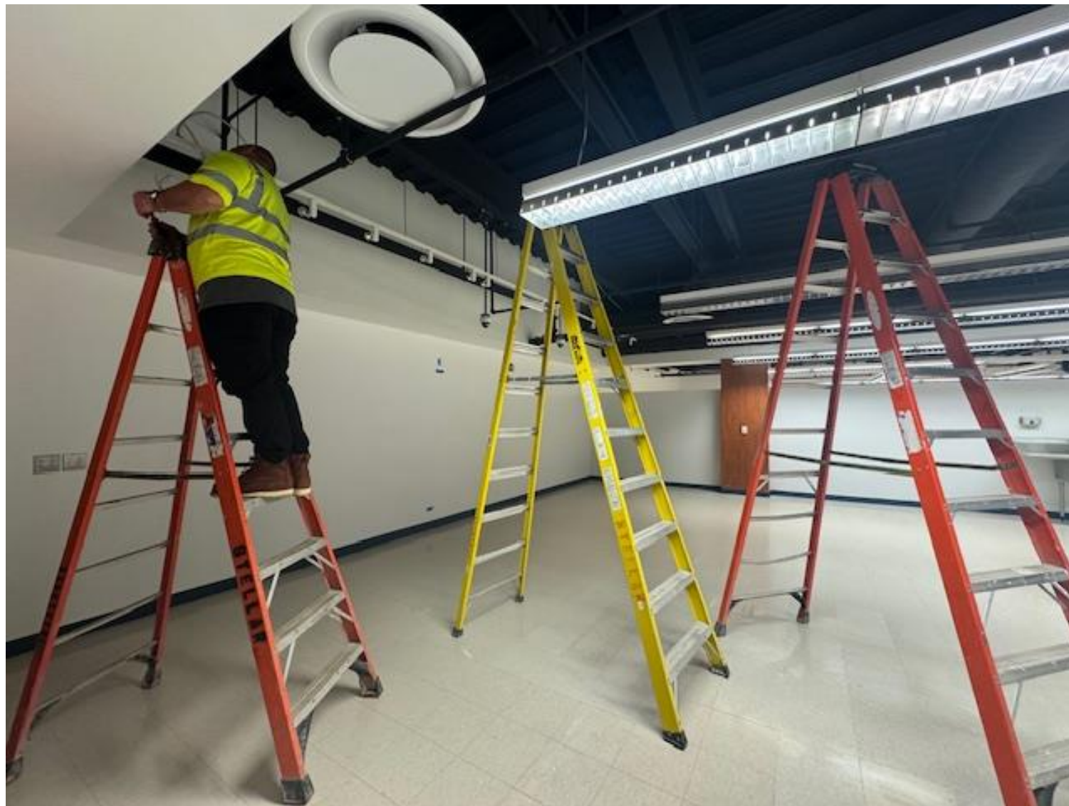
► Nursing Lab Renovation Project
