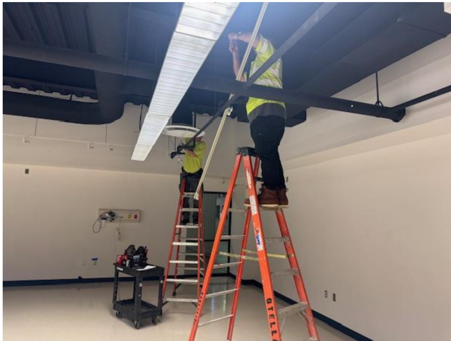
► Nursing Lab Renovation Project
