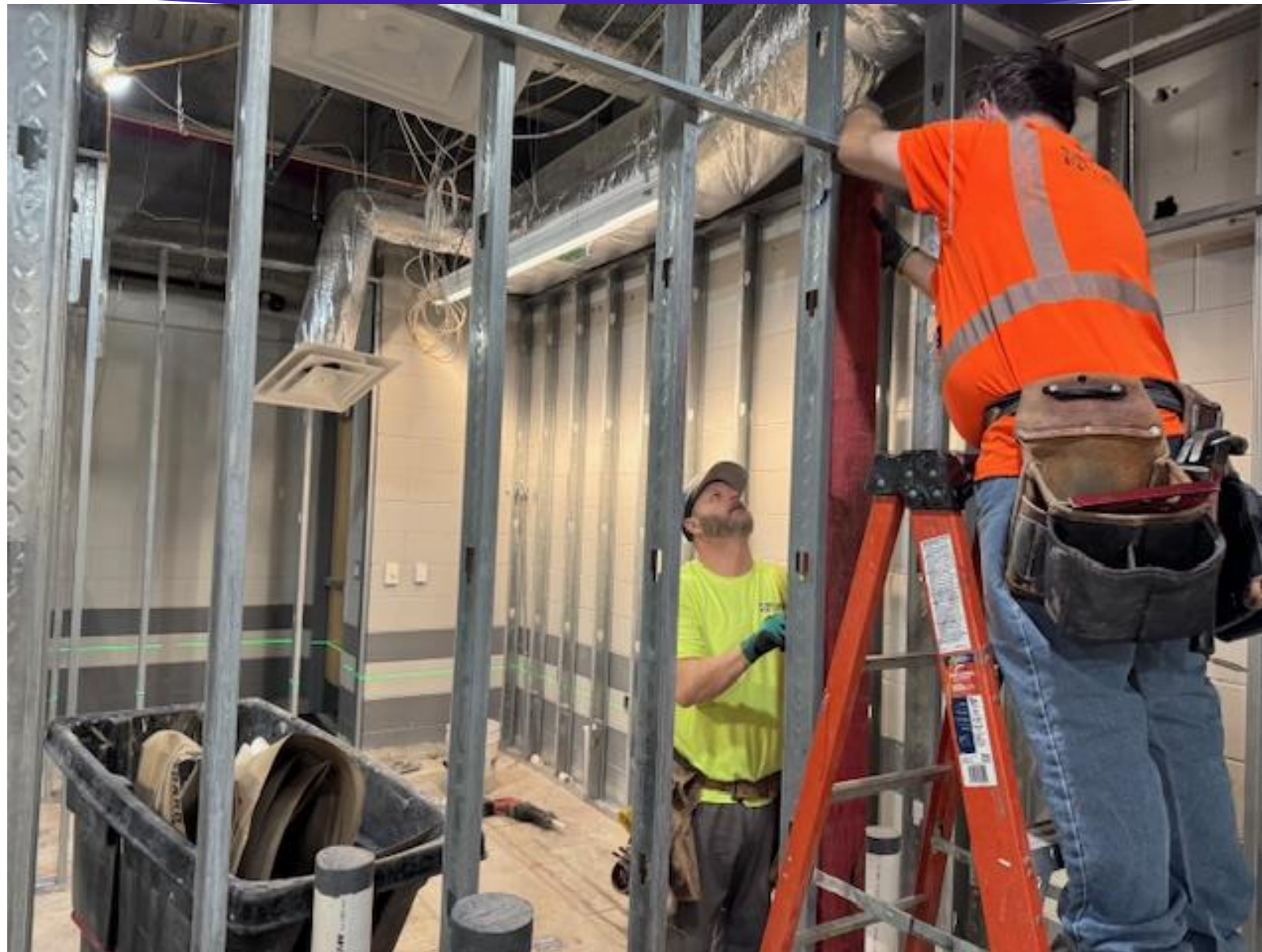
► Locker Room Renovation Project
