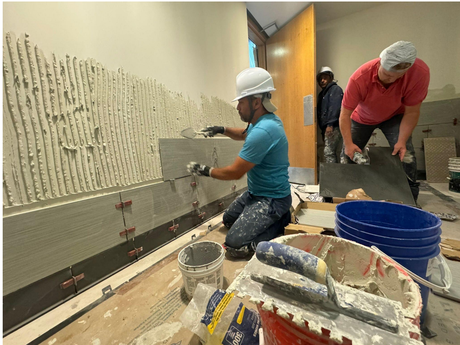
► Restrooms Renovation Project
